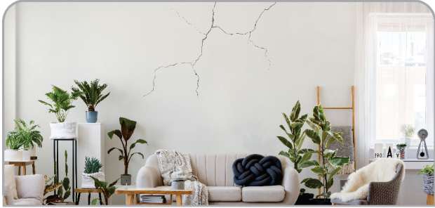
Cracks & Joints Filling
